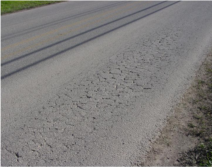
*Figure 1. Fatigue Cracking*
