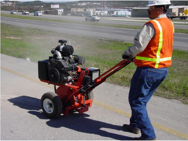
*Figure 8. Crack Routing Procedure*
