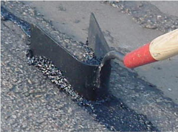
*Figure 11. Metal Finishing Squeegee for Use with Hot Pour Sealant*
